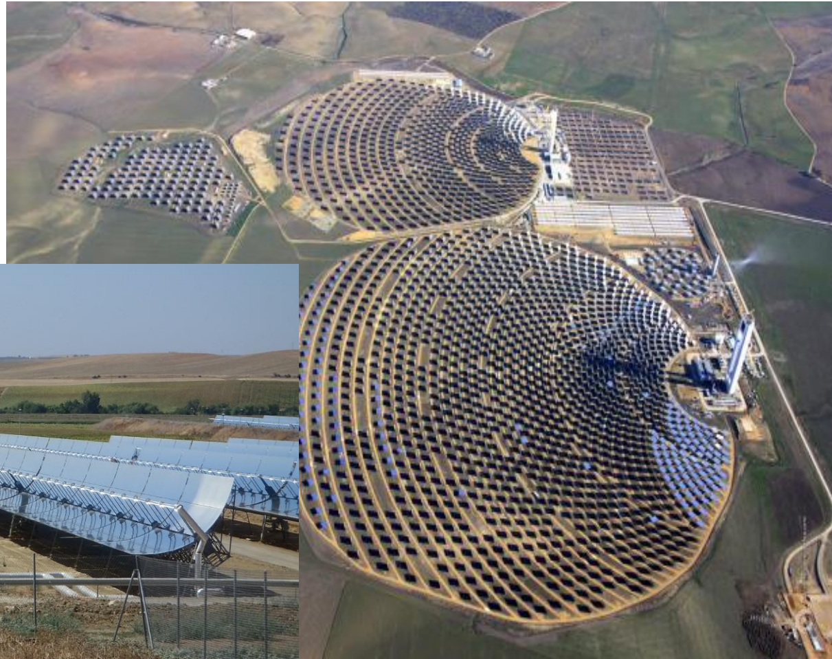
Pioneer thermosolar power plant. Sanlúcar (Sevilla) Spain (Abengoa)
